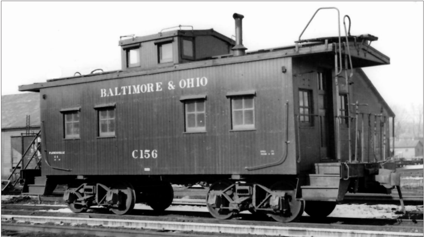
B&O C-156 - Freshly outshopped from the B&O shops at Painesville, Ohio, in late 1939, C-156 shows little modification from its as-built configuration. The underbody tool box has been removed and ladder grab irons have been added to the roof.
