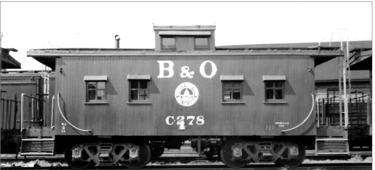
B&O C-278 - Last refurbished and painted at the Washington, Indiana, shops in June 1957, C-278 exhibits the 1955 to early 1960s lettering scheme. The car rides on Andrews trucks and exhibits the modified steps and end platforms which became standard on the B&O. The car also has the newer side grab irons and single-piece cupola window awning.
